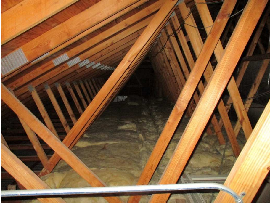
Roof Insulation over gypsum board plenum
