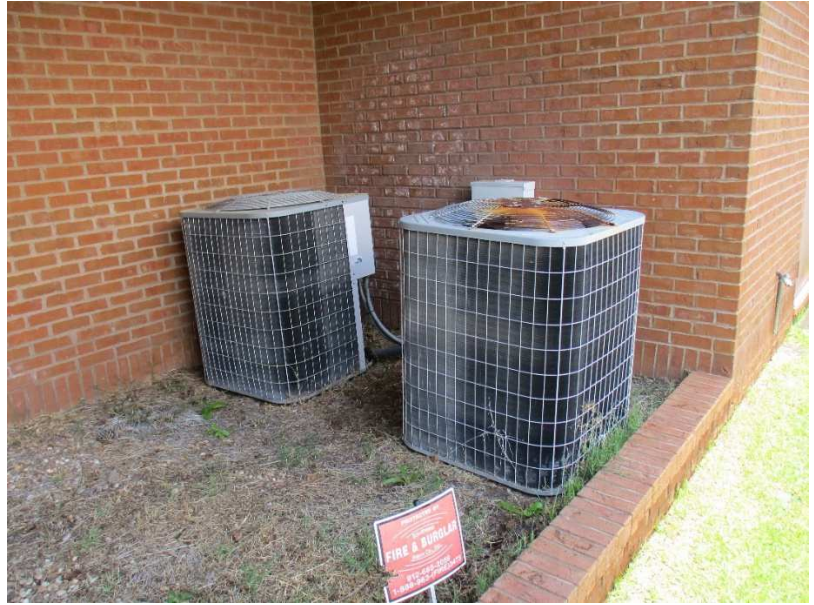
Multi-purpose room heat pump units
